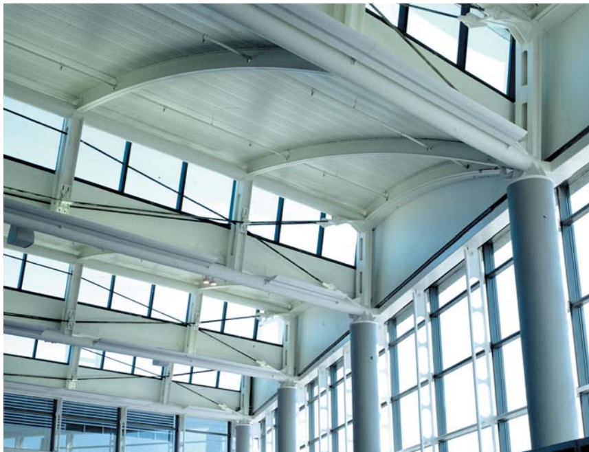
Continental Airlines, Terminal C, Newark International Airport, Newark, NJ Architect: Skidmore, Owings & Merrill Photo: Bruno Stieg, A/D Fire Protection Systems A/D FIREFILM® II on trusses and beams
