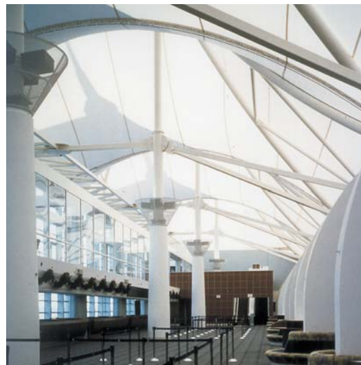
Royal Caribbean Cruise International Terminals 3 & 4, Miami, FL Architect: Bruno-Elias & Associates Photo: A/D Fire Protection Systems A/D FIREFILM® II on columns and beams
