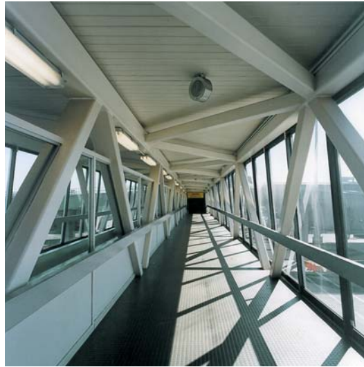
B.C. Ferry Terminal, Tsawwassen, BC Architect: Wade Williams Young Writers Architects in Joint Venture Photo: Alan Katowitz A/D FIREFILM® II on tubular trusses
