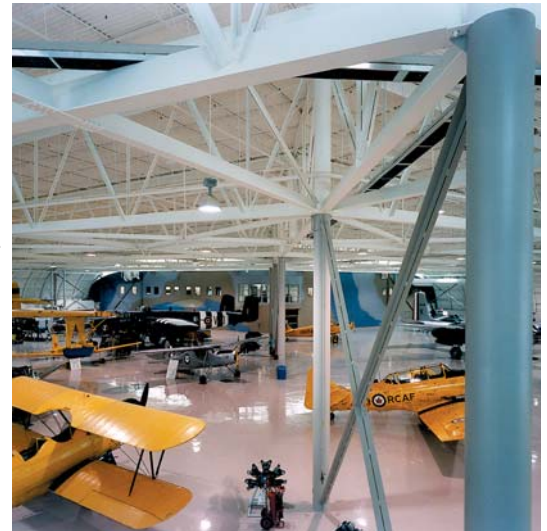
Canadian Warplane Heritage Museum, Hamilton, Ontario Architect: Chamberlain Architect Services Ltd. Photo: Lenscape Inc. A/D FIREFILM® II on tubular columns
